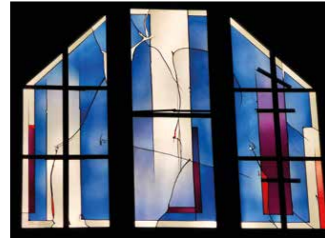
Project: window in our historic manufacturing hall
