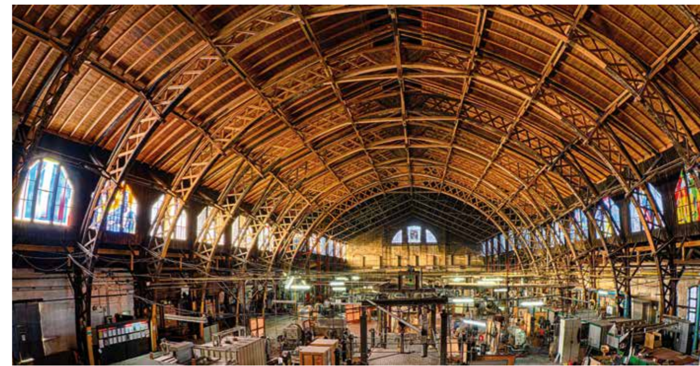
A look inside our furnace hall built in 1906.
