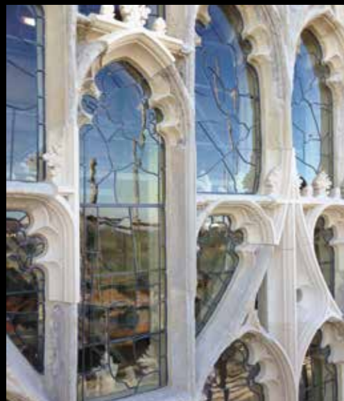
York Minster, Great East Window; Exterior protective glazing made of restauro® UV-protective glass as lead glazing
