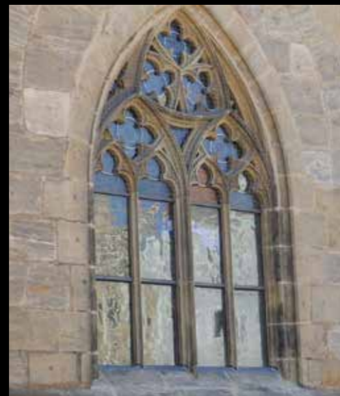
St Martin's, Amberg Mouth-blown window glass in the tracery thermally tempered; rectangular panes as laminated glass
