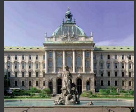
Palace of Justice, Munich, administrative and courthouse building from the late 19th century; restauro® ISO with restauro® Light 3mm; installation 2013/2014
