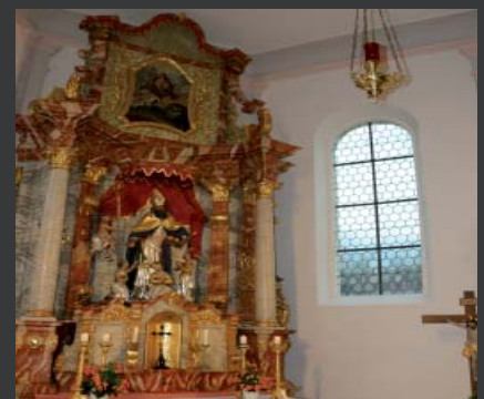
St. Nicholas Church, Wolfsbach/Bavaria; restauro®IR as honeycomb glazing to protect the baroque altar from the 18th Century; installation 2016
