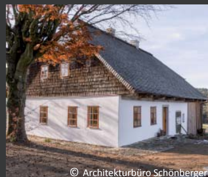
Waldlerhaus in Stadlern; one of the last typical farmhouses of the Bavarian and Upper Palatinate Forest; renovation distinguished with a monument award; window glazing consisting of restauro® ISO with restauro® Light 3mm in a 3-4-3 construction; installation 2016
