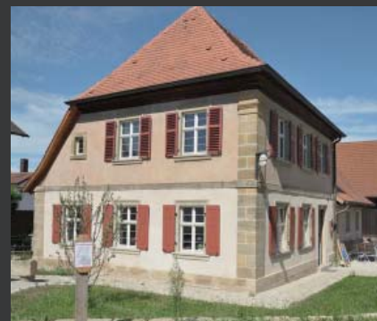
Historical building from the 18th and 19th century in Scheßlitz near Bamberg; restauro® ISO with restauro® Classic 3mm in a 3-10-3 construction; installation 2012
