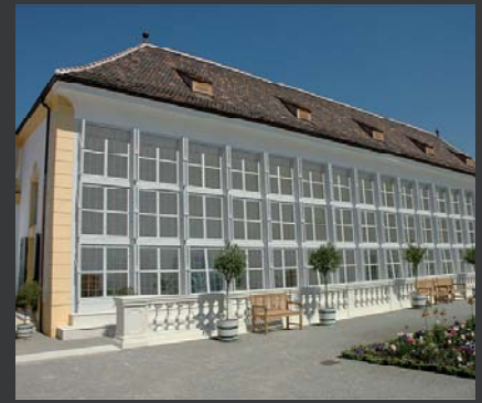
Orangery of Festschloss Hof near Vienna; window glazing with greenish restauro ® Waldglas in accordance with original glass fragments; installation 2006/2007
