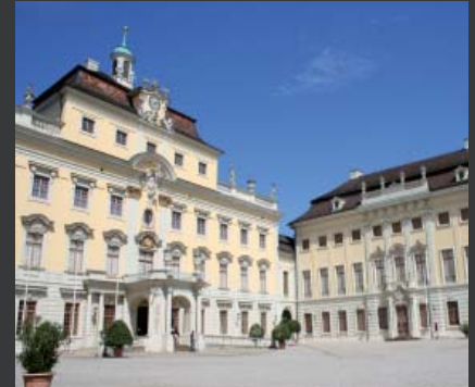
Ludwigsburg Residential Palace; built at the beginning of the 18th Century as a baroque castle; it served as the residence of the Duke of Württemberg temporarily; using restauro ® Light 2mm in the entire castle complex; renovation 1992-2004
