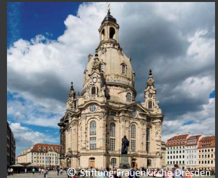
Frauenkirche Dresden; landmark, baroque monument building; destruction during World War II; reconstruction 1993-2005; installation of restauro ® Classic
