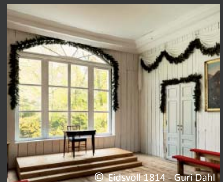
Eidsvoll Building, Eidsvoll (Norway); place of origin of the first Norwegian Constitution; window in the meeting room of the Imperial Assembly of 1814; using restauro ® Classic; installation 2013
